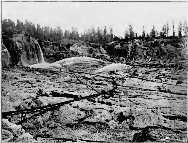
FIG. 139.—View in the Malakoff Hydraulic placer mine, North Bloomfield, California. From a photograph.
